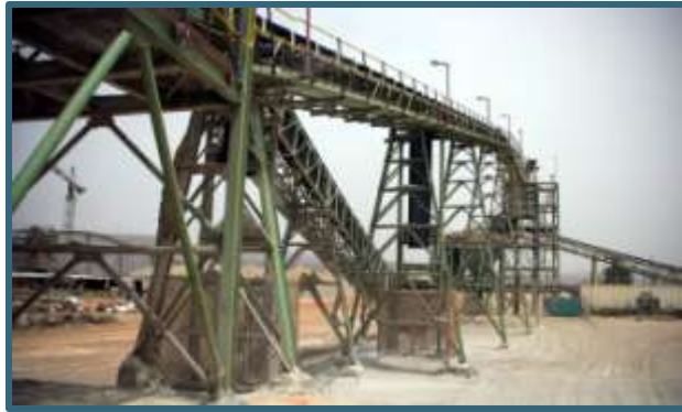
Milling Facility – 96% Au recovery
